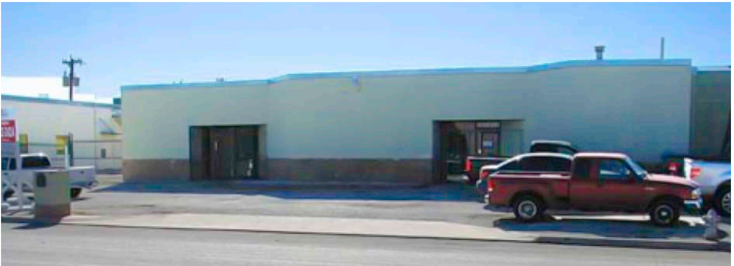
Front of Building
